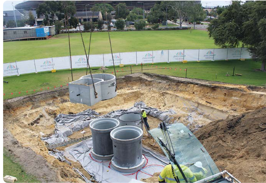
Construction of sewer pit and 3 overflow chambers to cope with high rates of usage.
