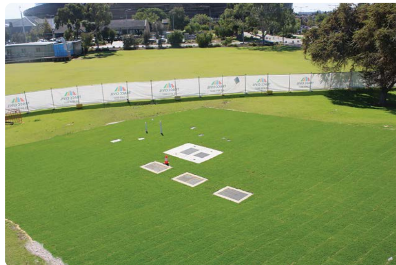
Completed sewer pit works.
